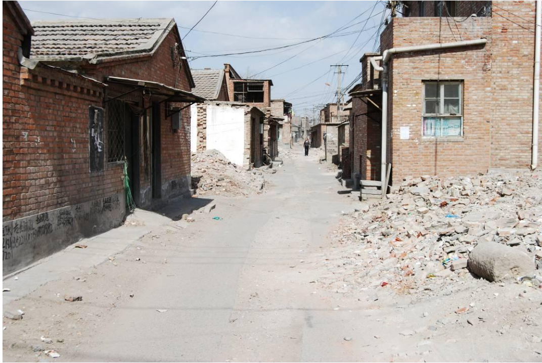
Photo 1: Partially demolished Shucun Village in 2008
